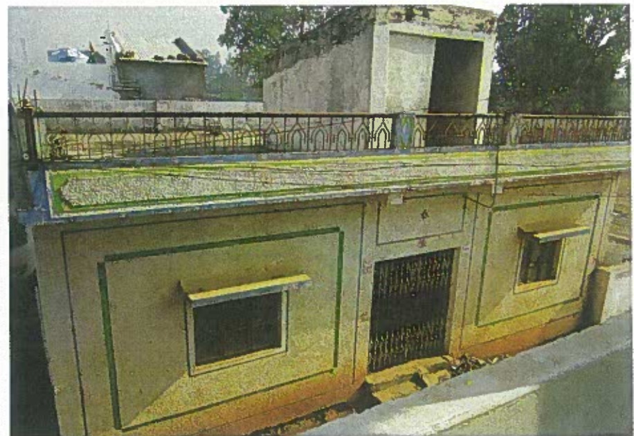
This building ground + 1 is typical example of projecting the main access as well as the rooms with projecting canopy as well as shaped chhajas which can allow the rain water to automatically slide and keep away from the face of the Building. Even the supporting window frame are segregated from the exterior plaster with grooves. The dividing column line of the Building stand segregated from the masonry work by grooves-so that the possible cracks are concealed.
